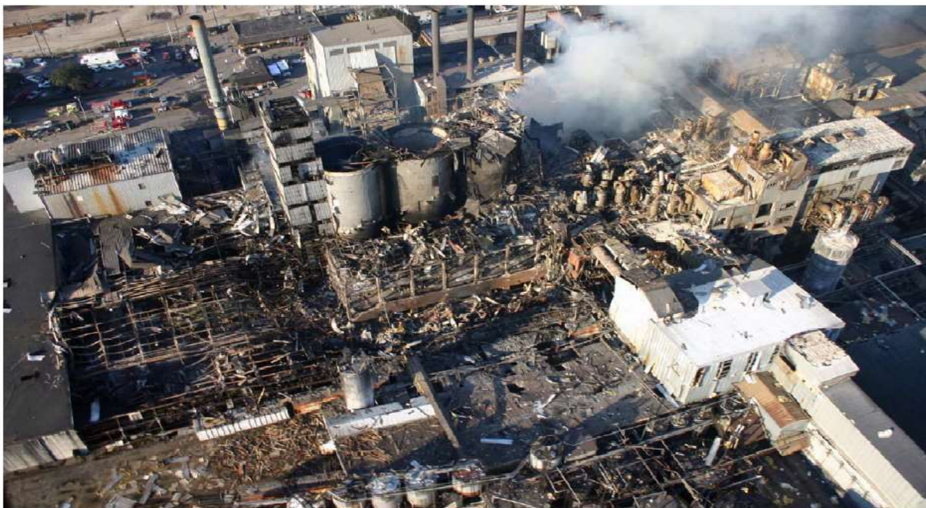
Figure 1. Aerial photograph of Imperial Sugar Port Wentworth facility after explosion.
