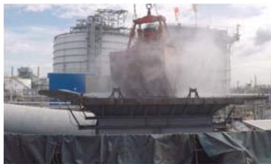
FOT. 3 Application of Freko-Humidifier integrated in customer’s installation
